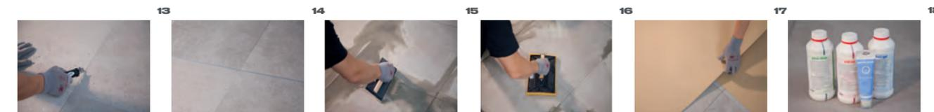
13- Prior to grouting, check that the bonding material has hardened. Remove the tile spacers, clean the joints along their length, width and depth, and check the joint is not damp.
