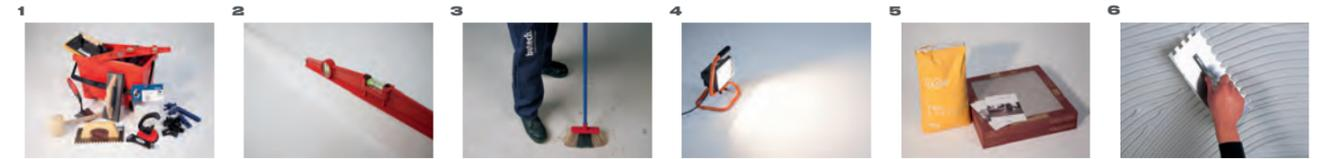
1- Installation of ceramic tiles should be carried out by skilled personnel, with demonstrable experience and appropriate tools and equipment, (i.e. toothed trowels, tile spacers, rubber mallets and suction cups for installation, and rubber trowels, sponges and containers for grouting). Check the information contained on the packaging beforehand, and meticulously follow the manufacturer's recommendations.
